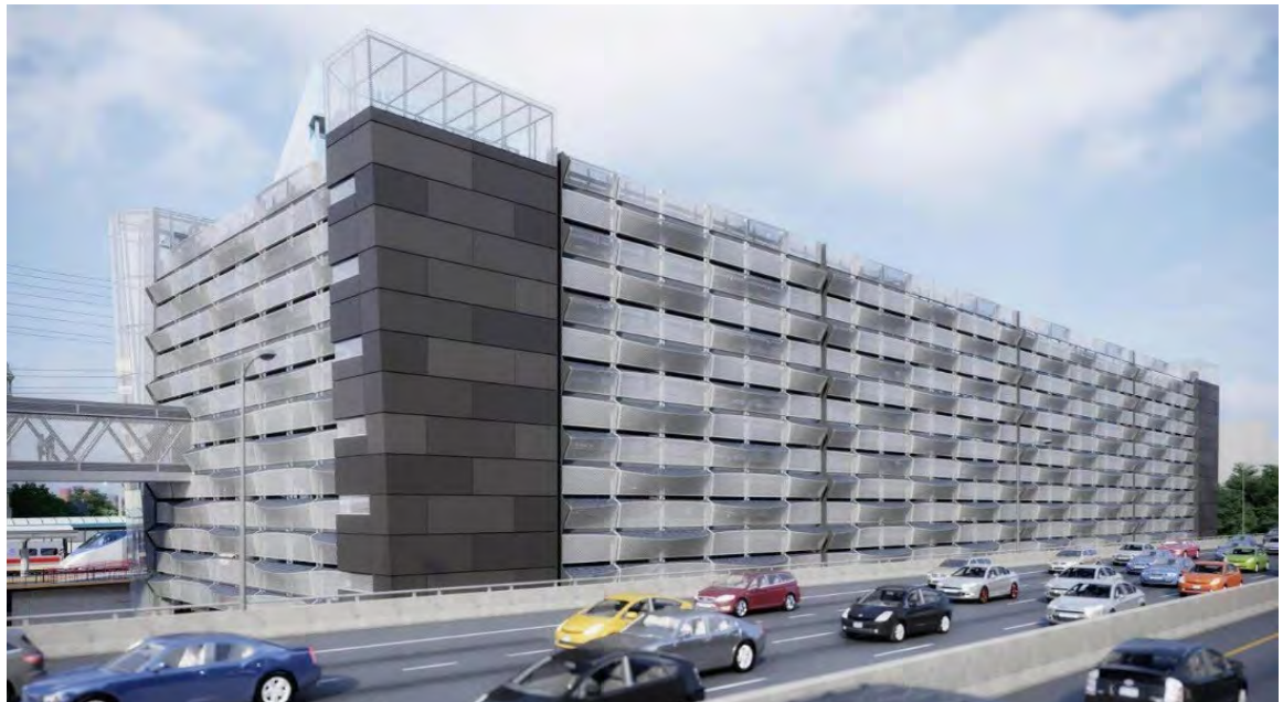
Figure 9: Stamford Station Parking Garage
